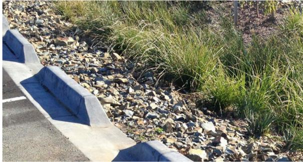
Raingardens are proposed around the site to provide storm water quality treatment for road and driveway runoff. The raingarden locations, size and design are to be determined based upon detailed design regarding site levels and drainage, but may include kerb inlets, as pictured.
